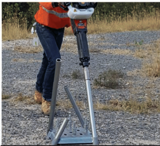
JACK HAMMER MICRO PILES
