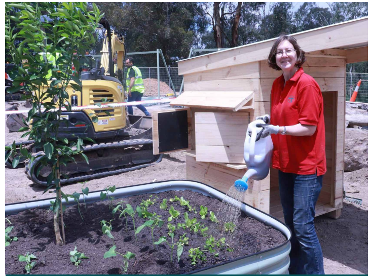
Rebuilding the Eltham North Adventure Playground
