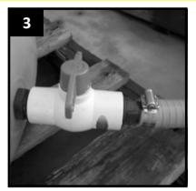
Screw one end of the Flexible Suction Hose onto the Ball Valve. (Check all hose clamps are fully tightened).
