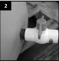
Connect the 25mm Ball Valve to the outlet of your rainwater tank.
