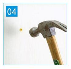
Insert the expansion screw into the drilled holes.
