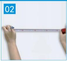
Measure the centre distance between the two hanging brackets and mark the corresponding position on the wall.
