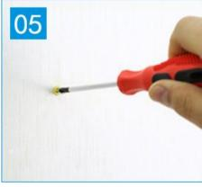
Drive the screw into the expansion screw, leaving 5mm out for hanging the mirror.
