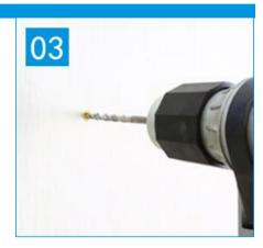
Use an impact drill to punch holes in the marked positions with a depth of approx. 5cm.
