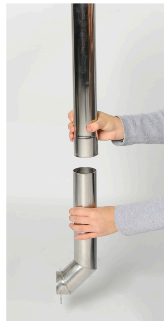
Lastly, connect complete flue assembly to the elbow bend or top of flue oven depending on configuration.
