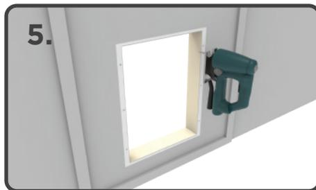
5. Using a reciprocating jigsaw, cut along marked lines.
