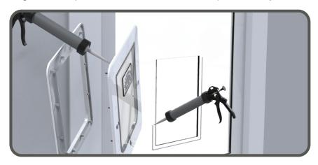
Refer to Steps 1 and 2 of "Installation". Place a bead of construction silicon around the internal section of the pet door and on the surface around the cut out to provide a weather seal. Tunnel is not required.
