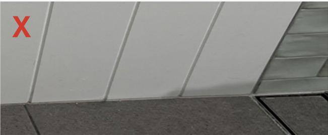
Panel used in a bathroom not installed on top of a skirting resulting in water wicking up the bottom of the panel and damaging it
