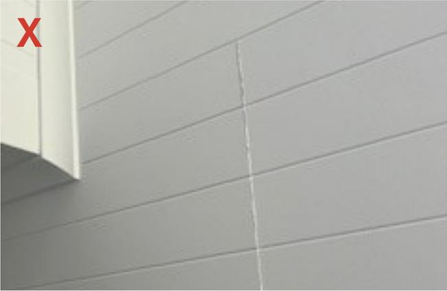
Panel joints showing when panels are installed end to end with no expansion gap or decorative trim cover
