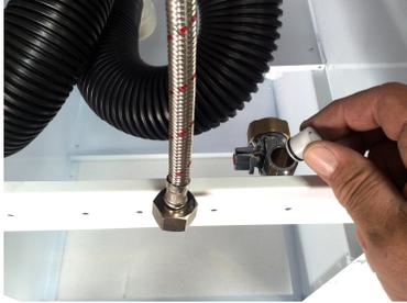
It is important to insert the valve **Spring** end first (left photo) as the valve only allows water to pass in 1 direction. Push the valve in until it is level.
