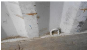
Example of tie-downs used throughout container
