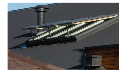
Pitched Roof Skylights
