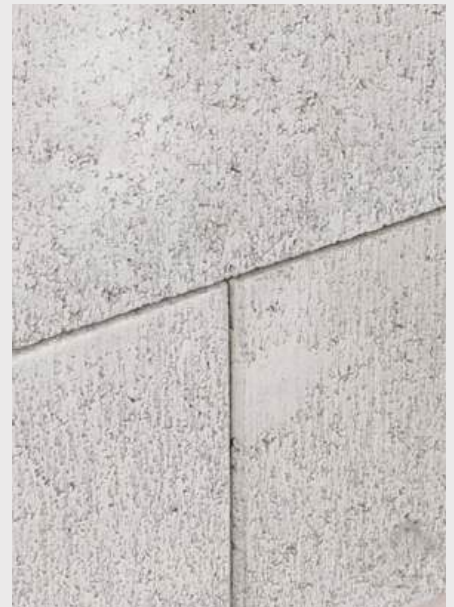
Clean wall with shadow lines
