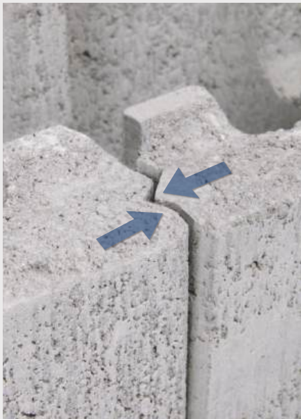
Interlocking tongue and groove joints
